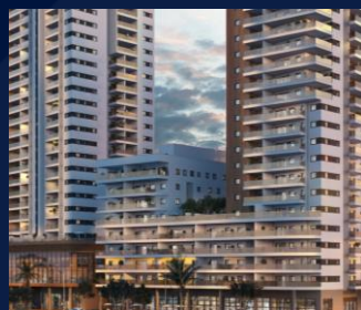
Ben Gurion, Ramla | Phase A | 270 housing units
